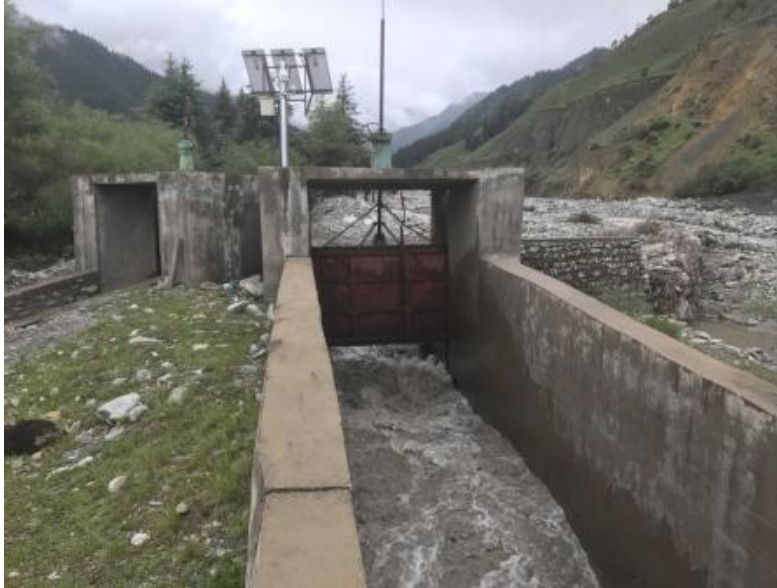
Fig. 19 Channels with Shallow Water and Washed-away Rocks
