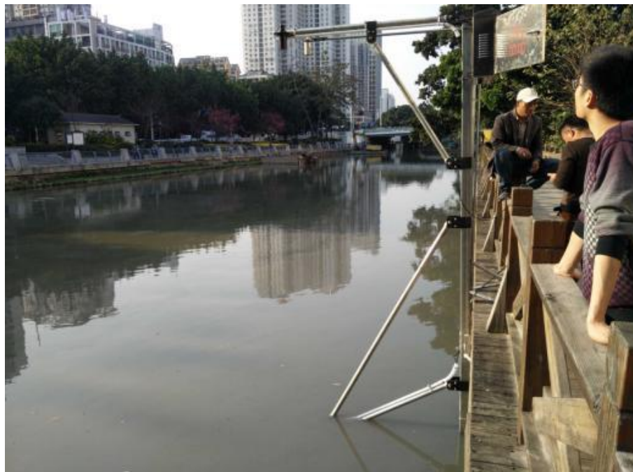
Fig. 31 Installation within River Channel
