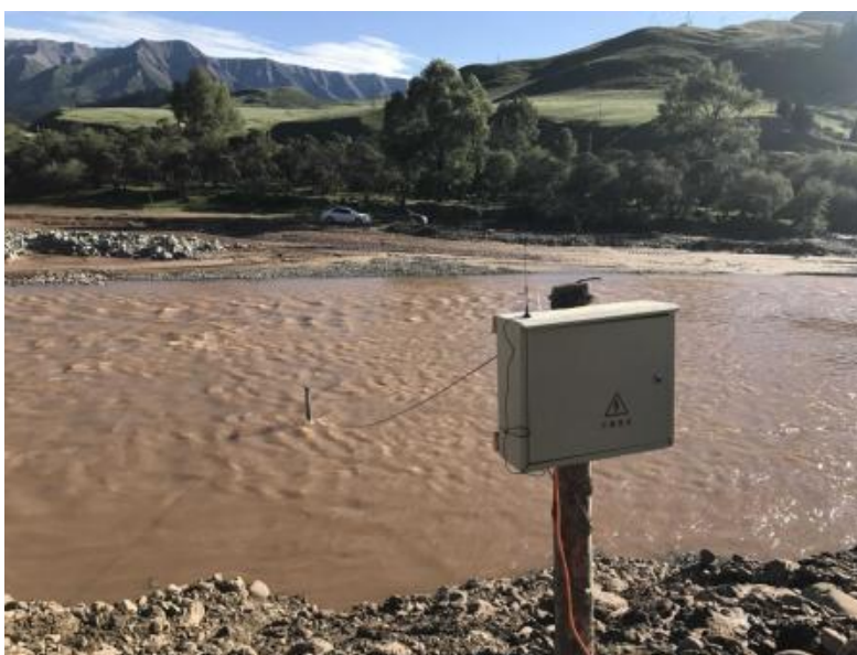
Fig. 19 Completed Installation in Wide River Channel
