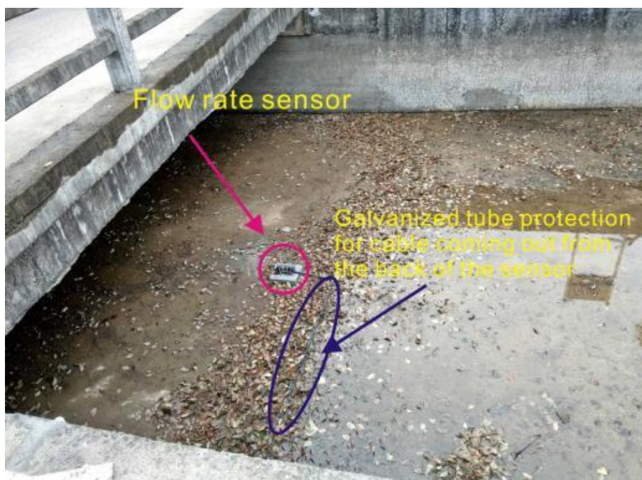
Fig. 20 Installation in Water Cut-off Channel
