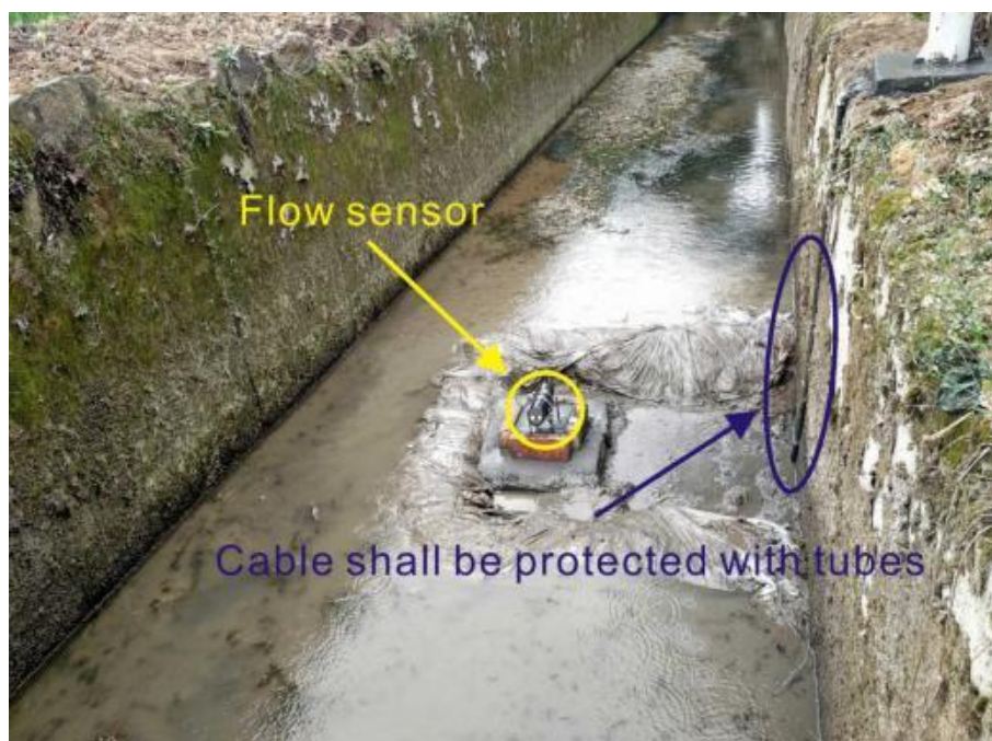
Fig. 27 Installation Mode for Channels with Silt Deposit
